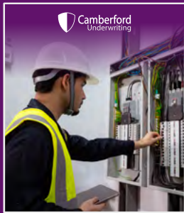
HVAC & Electrical Contractors
